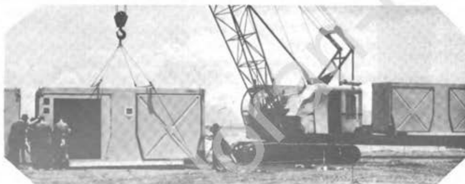
An ATLS shelter being positioned.
