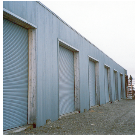
The only remaining WWII-era Army structure now used as a heavy equipment shed.
