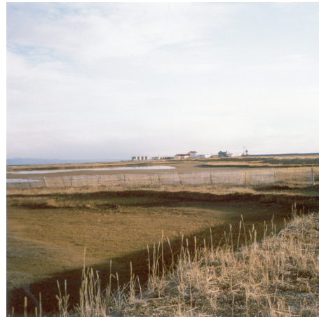
LORSTA Port Clarence with water supply ponds in the foreground.
