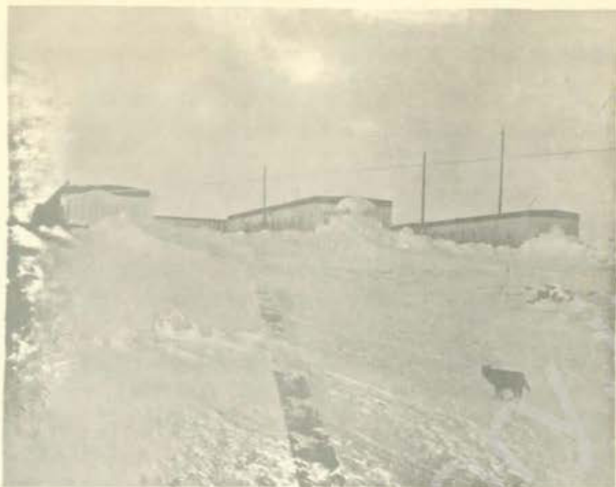
Station Building As Seen From The First Pump House Note utiliduct and Huskie in foreground
