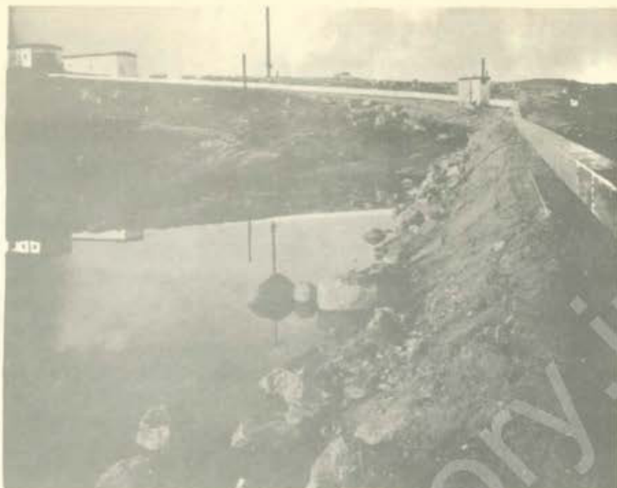
Reservoir and Utiliduct As Seen From The Second Pump House Road at right runs along the face of the dam. First pump house lies 128' from the water's edge.
