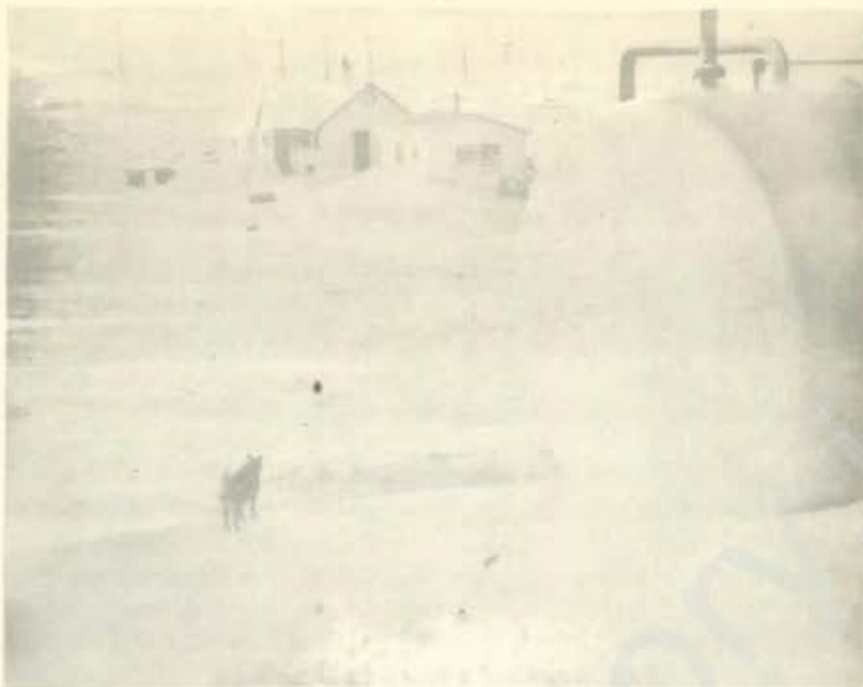
Royal Canadian Mounted Police Detachment Buildings One of five fuel oil storage tanks is pictured at right. Note Huskie in foreground.
