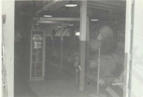
OLD ENGINE ROOM - JUNE 64
