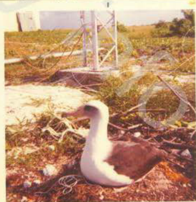
"GOONEY" AT BASE OF CONICAL MONOPOLE ANTENNA DURING DE-INSTALLATION.
