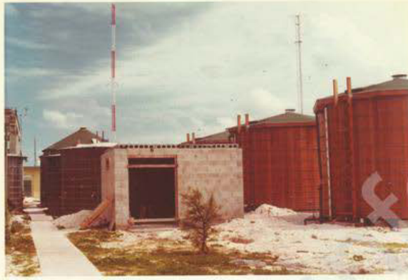
NEW WATER TANKS AND PUMP HOUSE NOVEMBER 1972 PHOTO BY ETC D. W. MENGE
