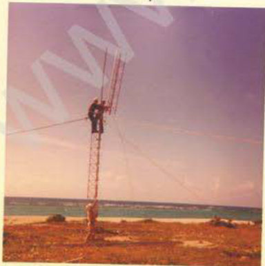
CWO NUZMAN, ET2 SCHRECK, ET3 DURHAM REMOVE CONICAL MONOPOLE ANTENNA THANKSGIVING WEEKEND 1973.
