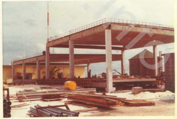
NEW S/P BUILDING NOVEMBER 1972 PHOTO BY ETC D. W. MENGE
