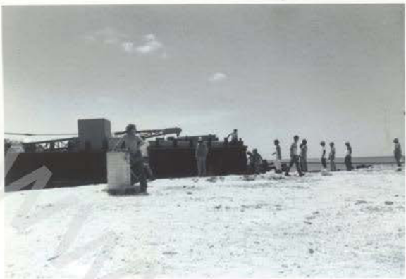
TUG MOHALA 10 JUNE 1972 OFF-LOADING REHAB SUPPLIES
