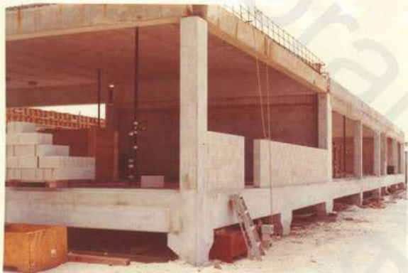
NEW GALLEY AND BARRACKS NOVEMBER 1972 PHOTO BY ETC D. W. MENGE
