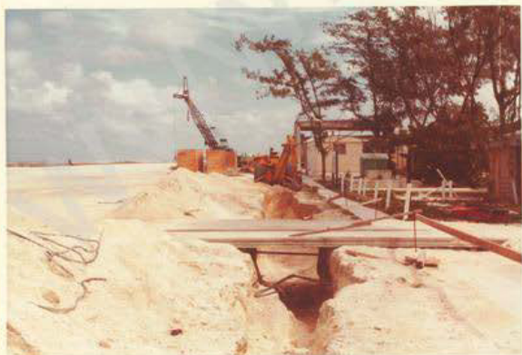
POWER AND WATER TRENCH NOVEMBER 1972 PHOTO BY ETC D. W. MENGE
