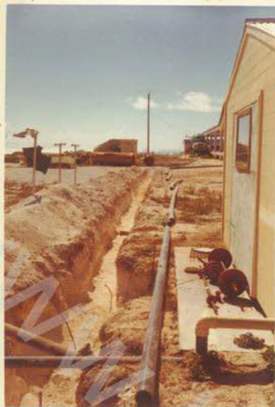
Station Rehab Oct 72
