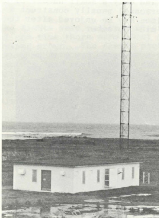
Transmitter building and 625-foot antenna
