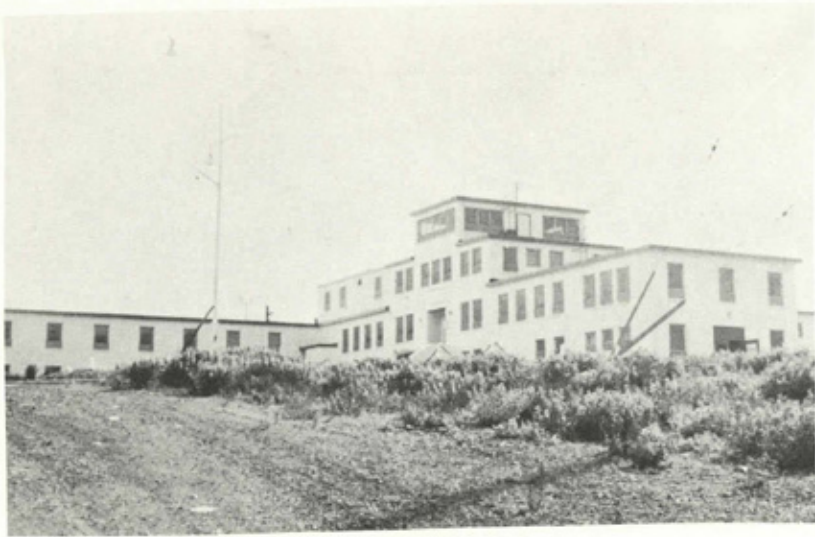
Station Building from Northeast
