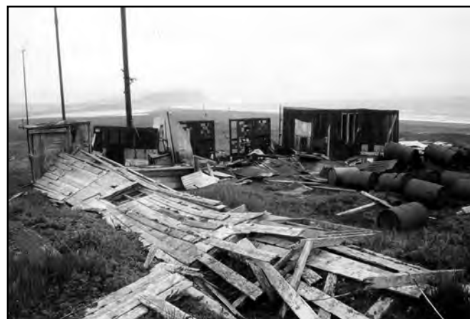
Figure 8: Loran A Station Quonset Hut and Tunnel, 2002.
