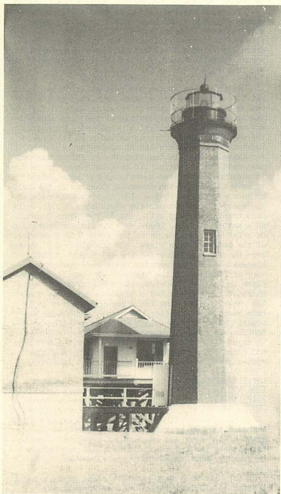
ARANSAS PASS LIGHT STATION, PORT ARANSAS, TEXAS
