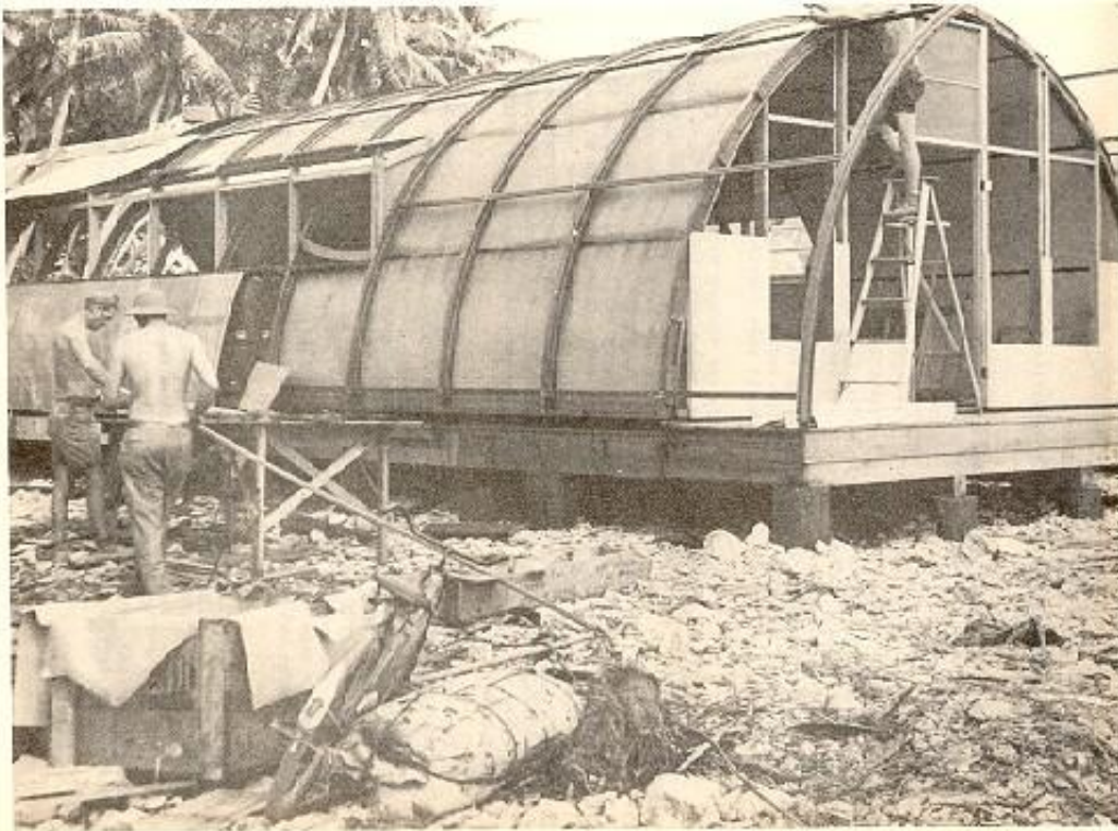
STEEL FRAME AND INTERIOR SHEATHING OF A QUONSET HUT
