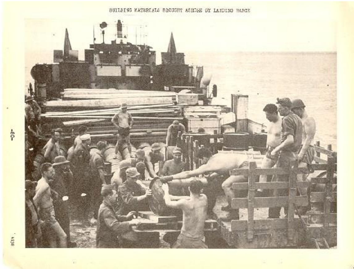
Image Caption: BUILDING MATERIALS BROUGHT ASHORE BY LANDING BARGE
