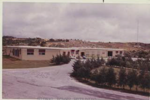
SIGNAL TOWER BUILDING
