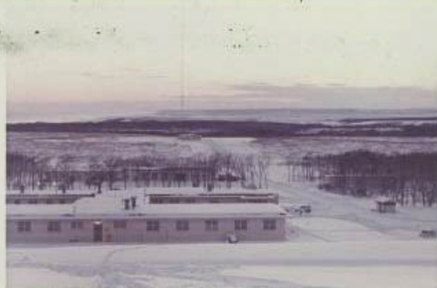
STATION VIEW FROM HELICOPTER PAD
