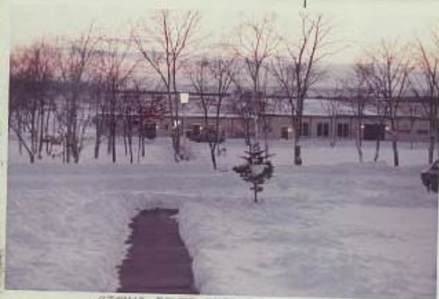
SIGNAL POWER BUILDING AT DUSK
