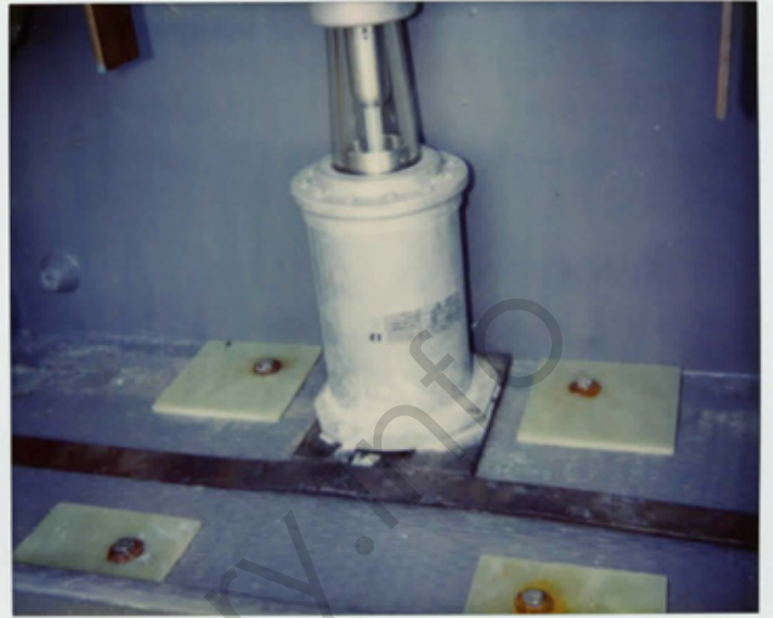
Lightning arrester between tower, station
