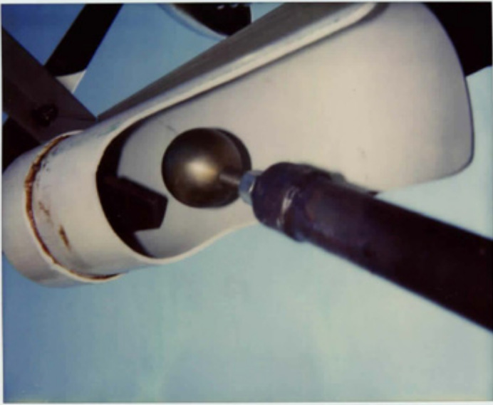
Tower Z-Feed spark gap
