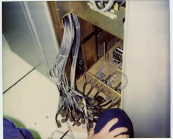
Cables to SDA, SDA removed, inside view of CPS
