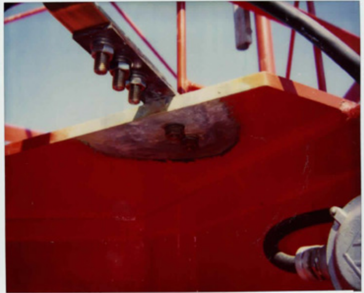
Pri transmission line to tower point of connection with Z-Feed from X-mtr hooked up
