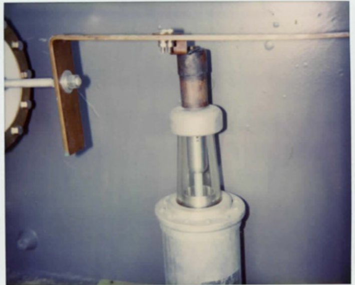
transmission line, lightning arrester between tower, station
