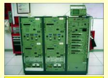
Figure 4. AN/FPN-54 Timing Rack where the LORAN pulses are generated for amplification in the AN/FPN-45 vacuum tube transmitter. Photo courtesy of ETC K. Anderson.
