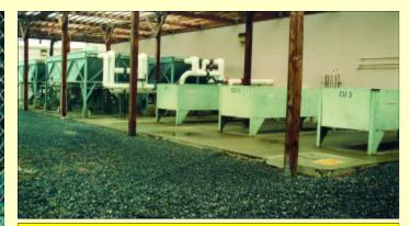
Figure 11. This is what it takes to remove the heat from the transmitters. The A/C units are rated at 30 tons each. There are four heat exchangers (HEX) to cool the deionized water used for the driver/PA tubes. Photo courtesy of ETI K. McKinley.
