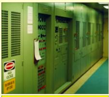
*Figure 6*. One of the two AN/FPN-45 transmitters on air, cranking out 1.6 megawatts.
